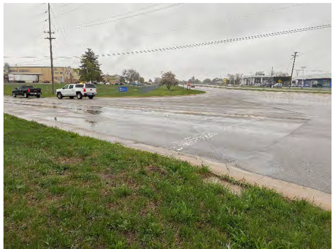
FIGURE 5. Photo looking southward at the Howell Road / Cedar Street intersection.
