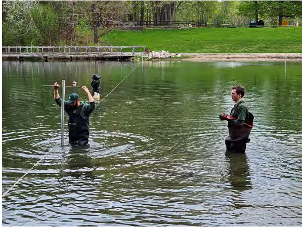
Swimming Beach Install
