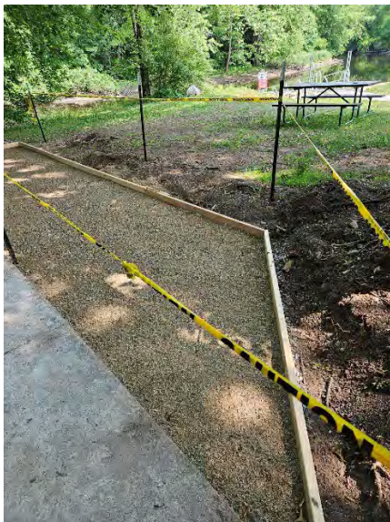
Concrete Pad Prep Work
