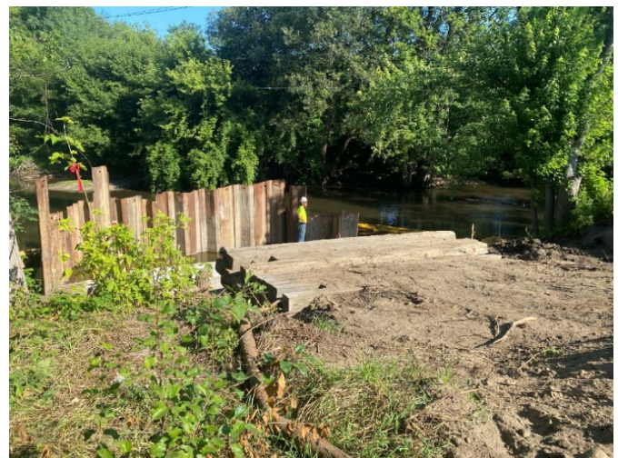
Contractor pulling out sheet piling
