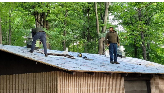
Park Staff Repairing Skylight Openings
