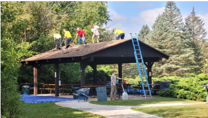
Trumble Construction Crew Removing Shingles
