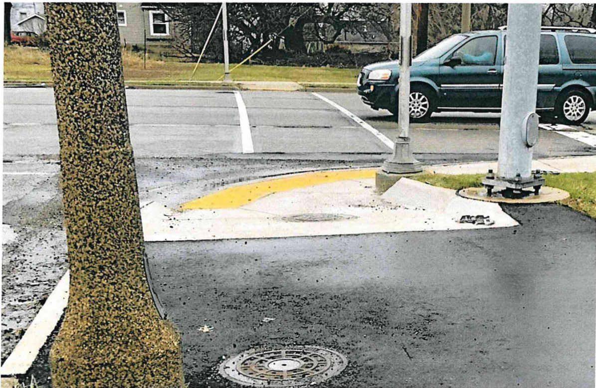
Looking North at the Grand Avenue/Oakland intersection: constructed ADA ramp
