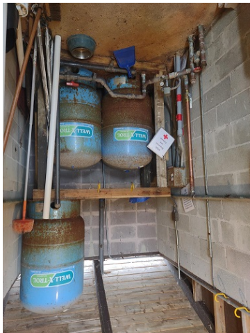
Pressure tank replacement
