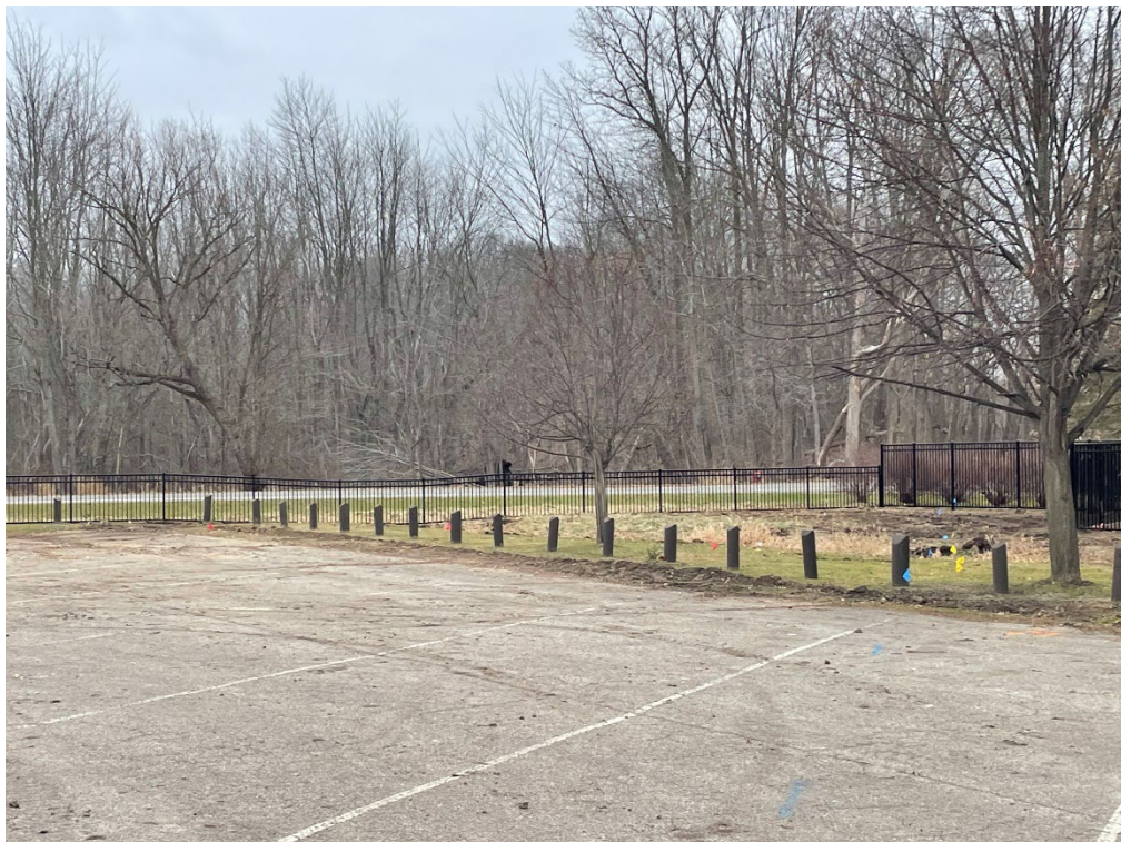
Lake Lansing Boat Launch renovation new fencing
