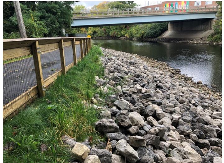
TR038 Washington Avenue: HMA, Rip Rap plantings and Rail repair
