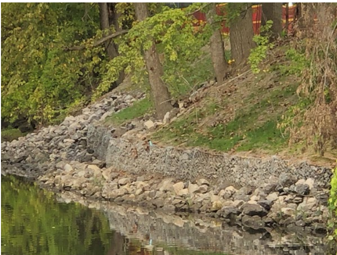
TR029 Grand River N Section: Rip Rap, Gabion Basket and slope restoration
