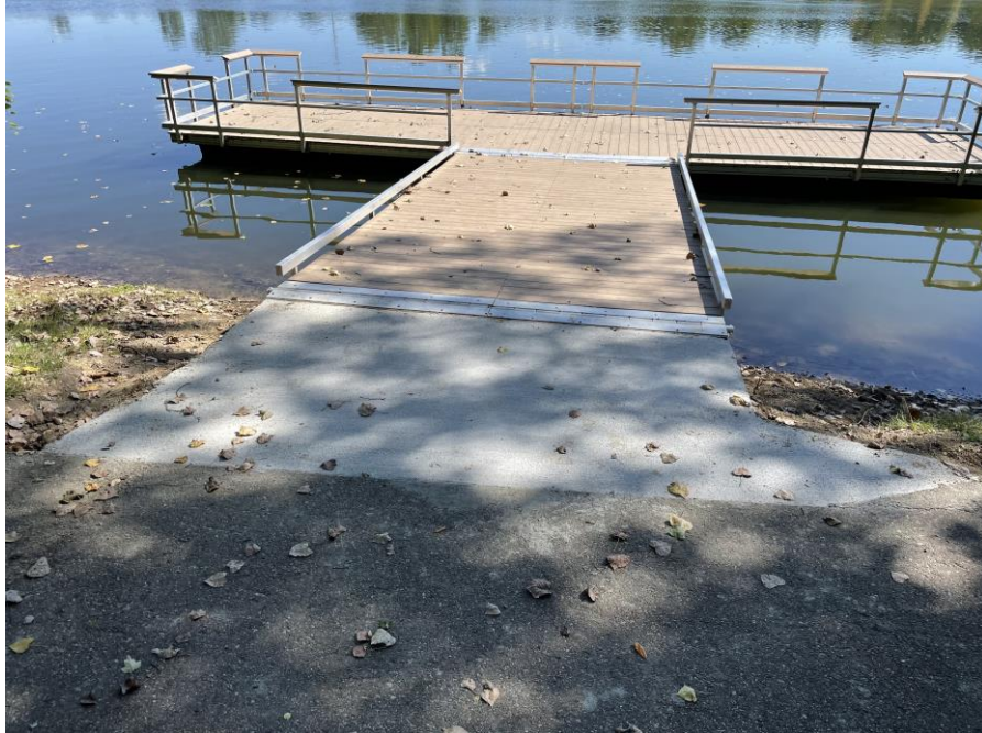
New accessible concrete transition onto fishing docks
