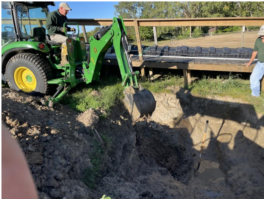
Staff digging down to attach snow making pipe hydrants
