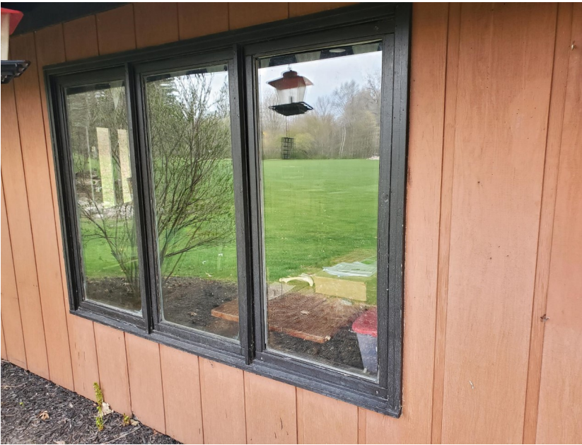
Replace casement windows with 2 pane insulated windows
