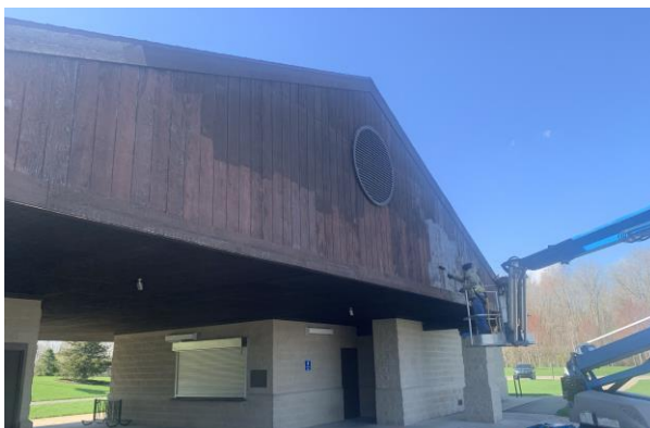
Re-staining of Northern gable face of Beach House building
