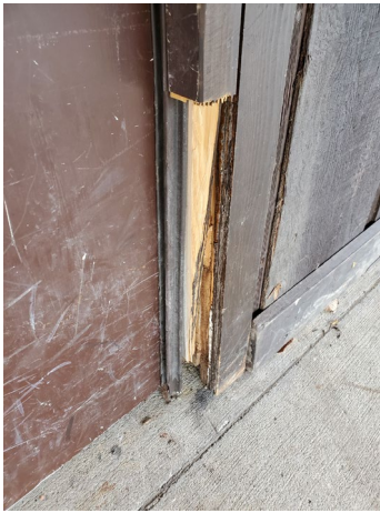
Some of the damage to doors and panels from installing year after year.
