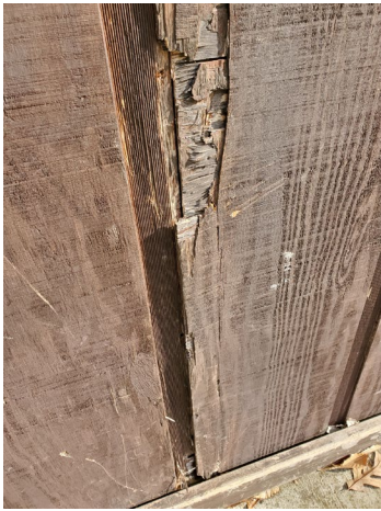
Some of the damage to doors and panels from installing year after year.
