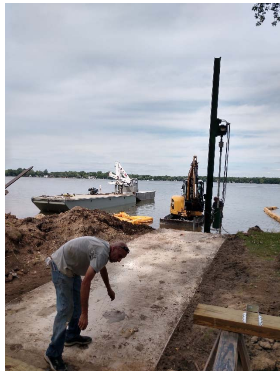
Concrete abutment for new dock
