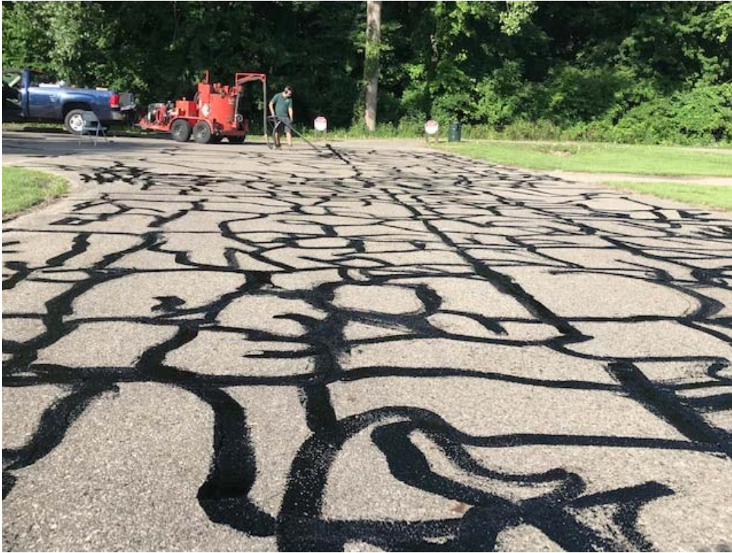
Crack Sealing Beach Parking Lot at Hawk Island
