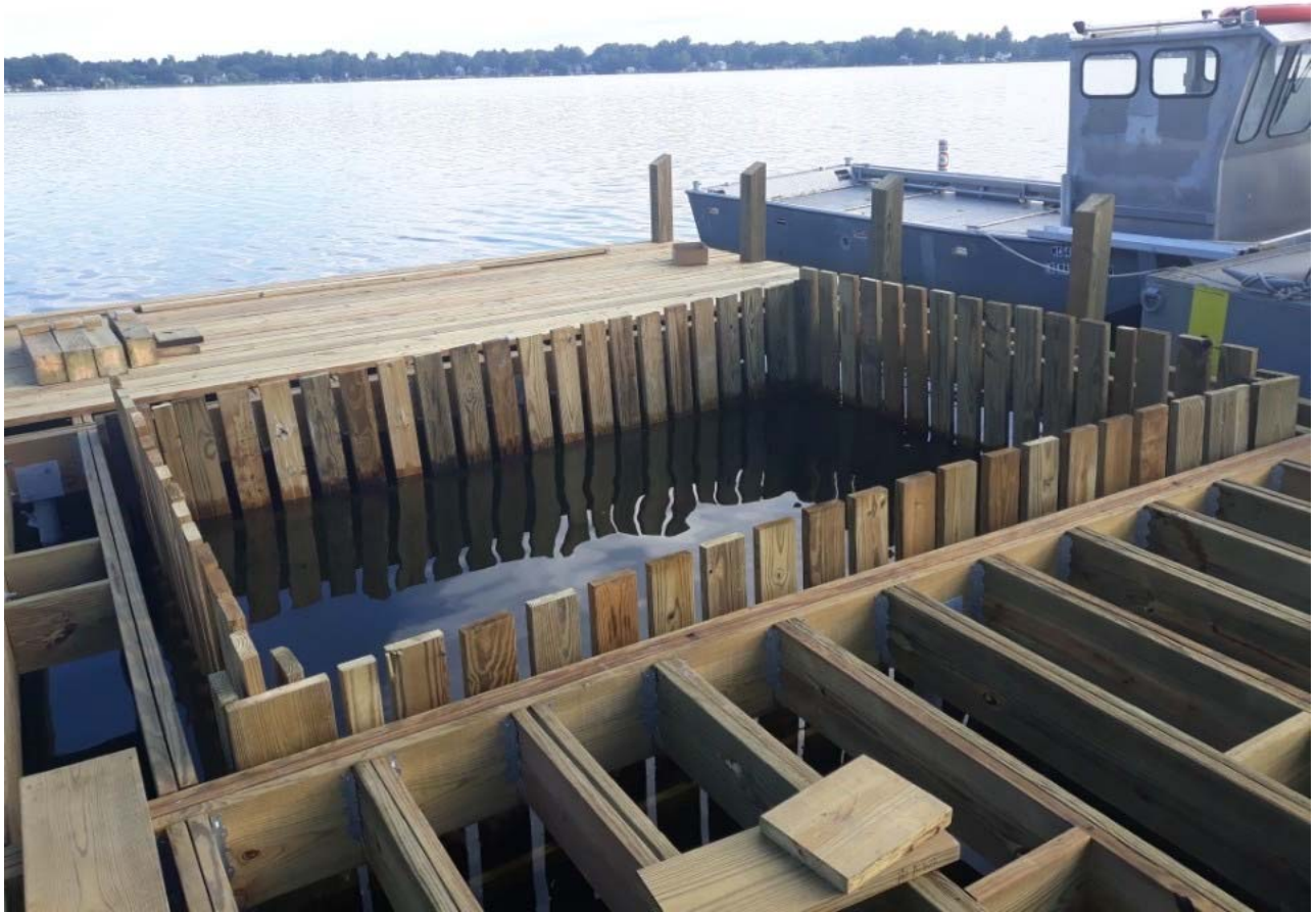
Photo of new fish habitat cribbing being added prior to decking for Lake Lansing South new Dock/Fishing Pier!
