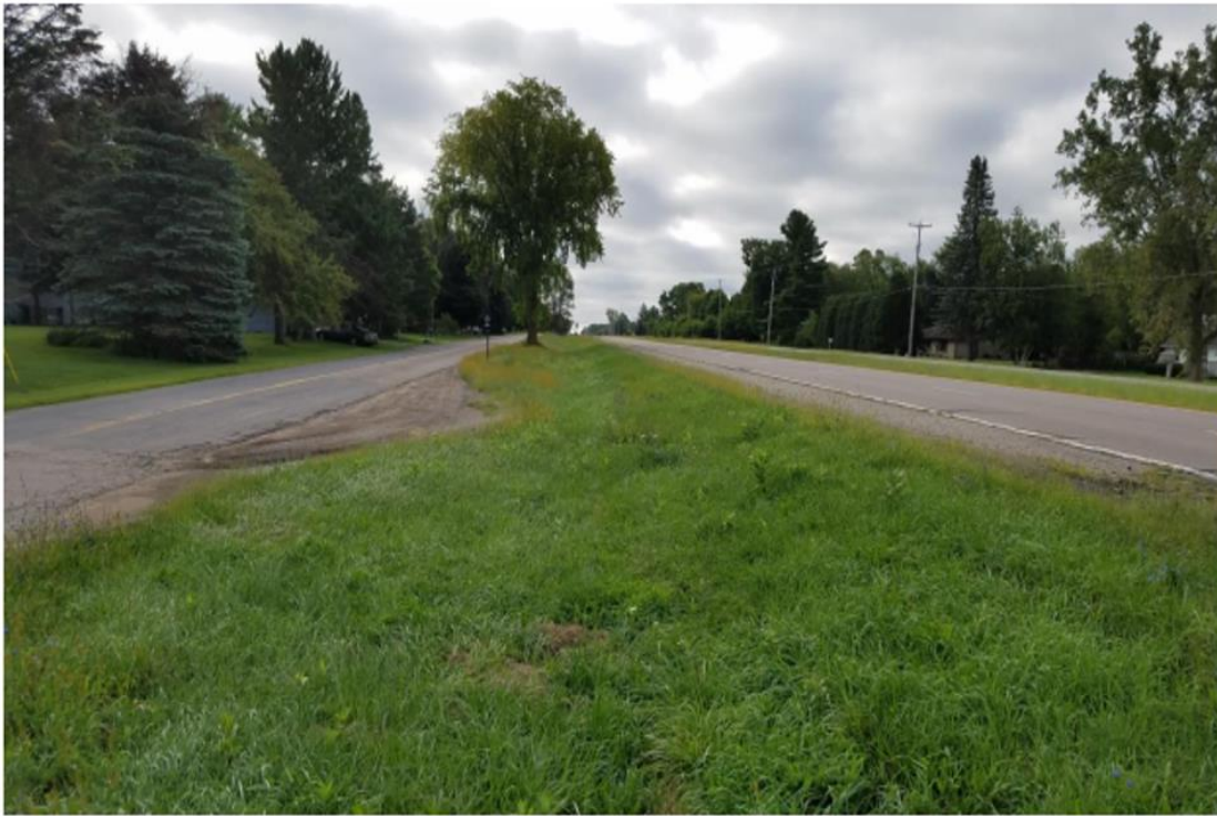
Photo 8. Typical Ditch to be Filled and Replaced with Underground Stormwater, Looking South (Hogsback Rd is on the left)
