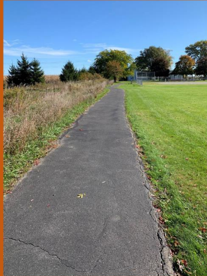
White Oak Township 2011 Trail Asphalt over Topsoil
