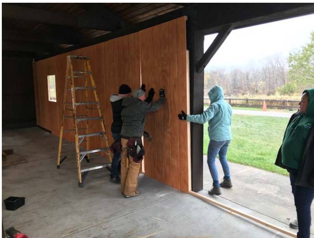
Installation of new wall panels at Red Tail Shelter
