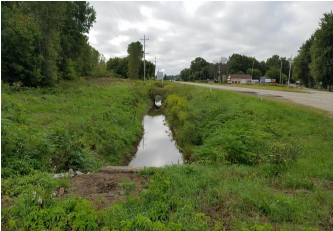
Photo 5. Typical Ditch to be Filled and Replaced with Underground Stormwater, Looking South
