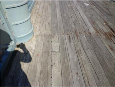
Typical bridge decking
