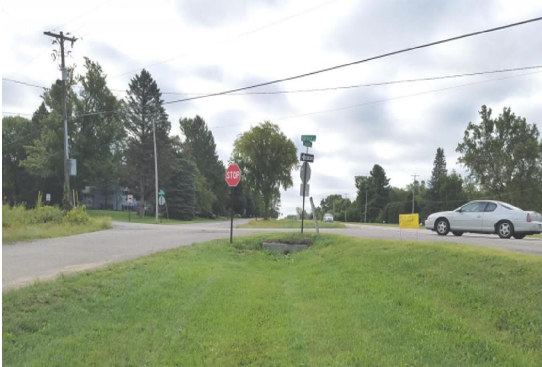
Photo 7. Future Crossing at Harper Road, Looking South (Hogsback Rd is on the left)
