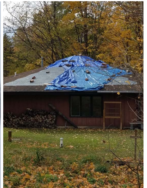
WSB roof replacement
