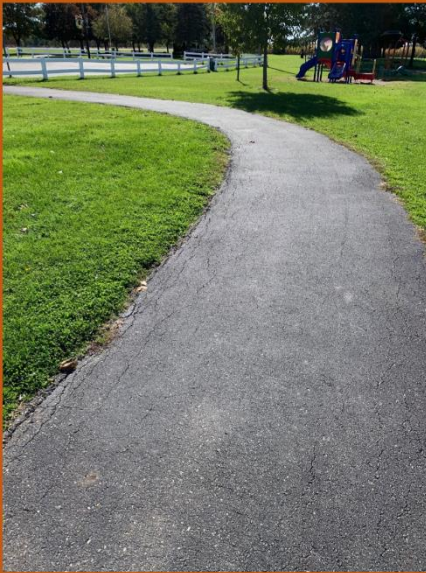
White Oak Township 2011 Trail Asphalt over Topsoil
