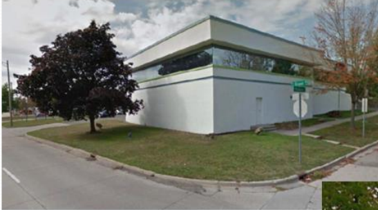
Grand Avenue at Madison Street looking at the southwest corner where the sidewalk currently terminates. The sidewalk will be extended to connect to the pathway proposed on the east side of Grand Avenue.
