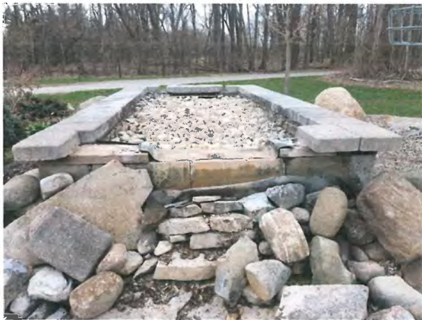
Hole #18-Waterfall needs new rubber liner and rock
