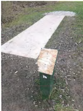
T-Signage starting to separate
