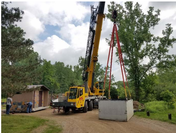
Setting the concrete pit toilet building at Mac
