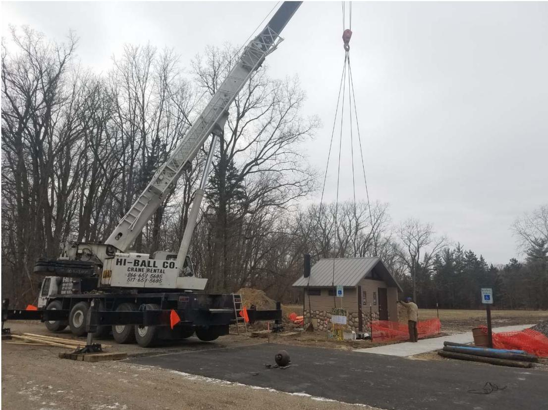
CXT restroom building being installed near Overlook shelter.
