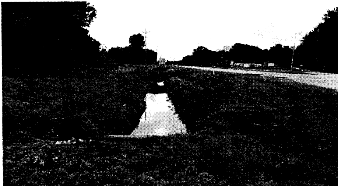
Photo 5. Typical Ditch to be Filled and Replaced with Underground Stormwater, Looking South
