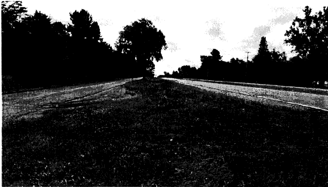
Photo 8. Typical Ditch to be Filled and Replaced with Underground Stormwater, Looking South (Hogsback Rd is on the left)
