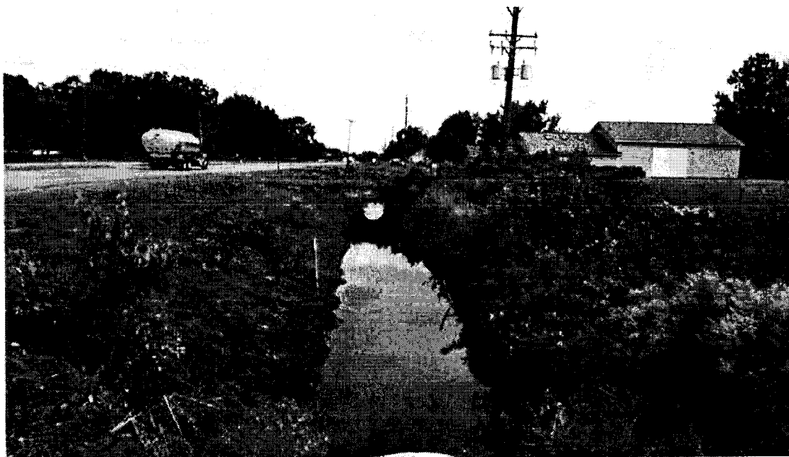
Photo 6. Typical Ditch to be Filled and Replaced with Underground Stormwater, Looking North
