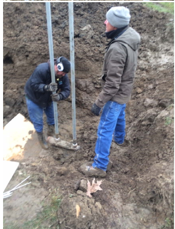
REPAIRS TO MAIN SNOWMAKING LINE AT HAWK ISLAND
