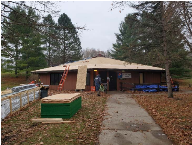
New decking on WSB roof
