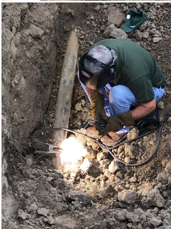
REPAIRS TO MAIN SNOWMAKING LINE AT HAWK ISLAND
